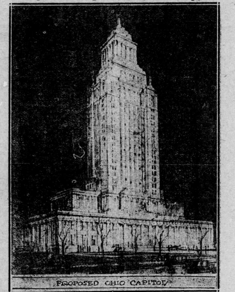
This proposal for increasing the office space in the Ohio State Capitol, at Columbus, has been approved by a special committee of the Legislature, and is likely to be formally adopted when the Legislature meets this Fall. The present Capitol constitutes what is the lower flat structure in the above picture. The central tower would be constructed in the courtyard of the present building and provide facilities for the State for years to come.
