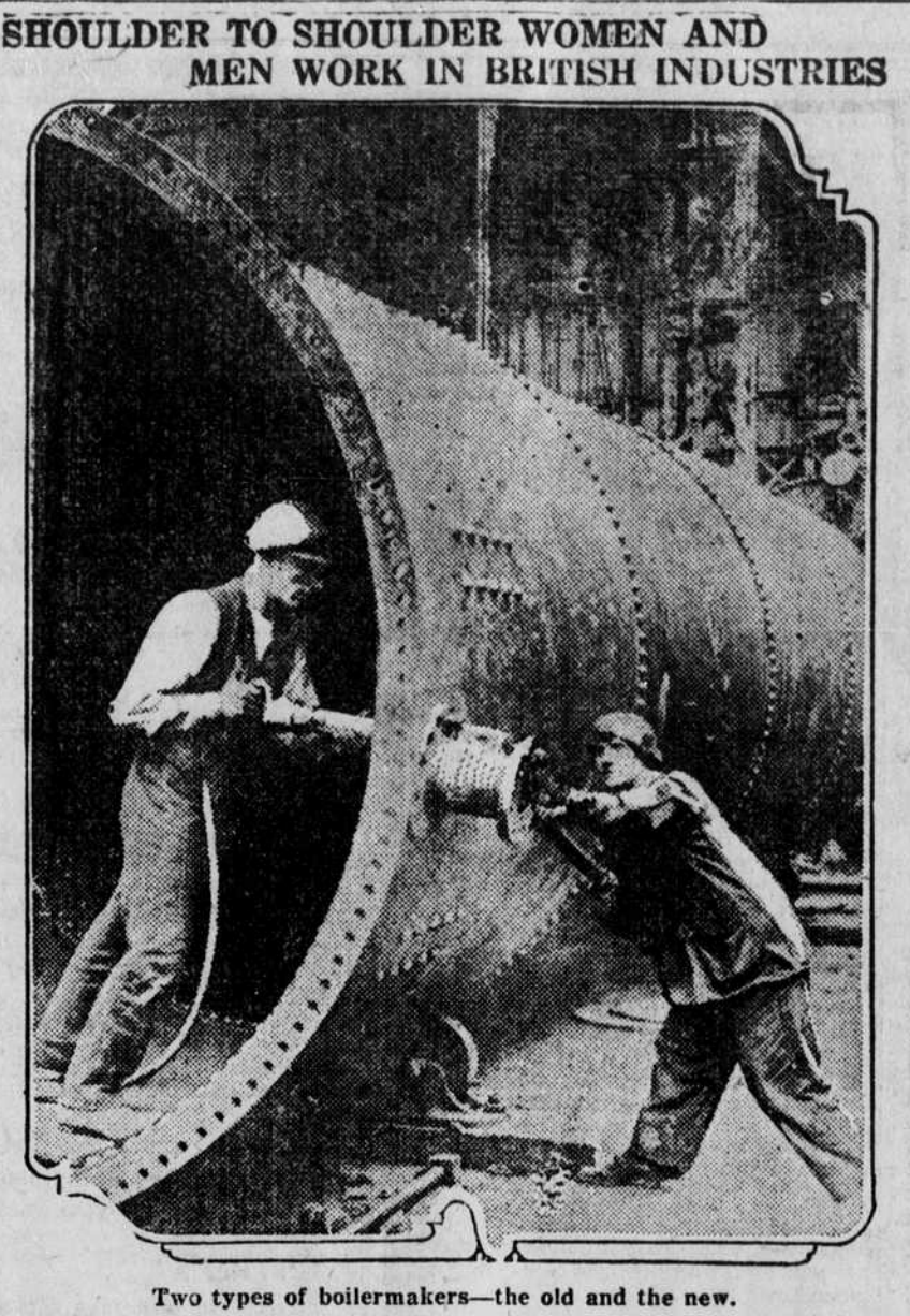
Two types of boilermakers—the old and the new. As a rule boilermakers are not considered ladylike, but this plucky woman has thrown tradition to the winds and entered on a career in a boiler factory in Glasgow. Clad in working togs deserted by a huskier boilermaker when the call to the colors sent him to the front, she is shown in this picture working a hydraulic riveter, assisted by a man.
