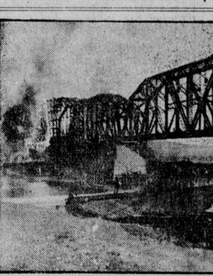
BIG RAILROAD BRIDGE AT MOBRIDGE, S. D.
