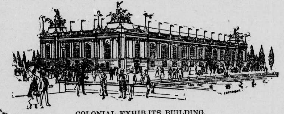
COLONIAL EXHIBITS BUILDING.
