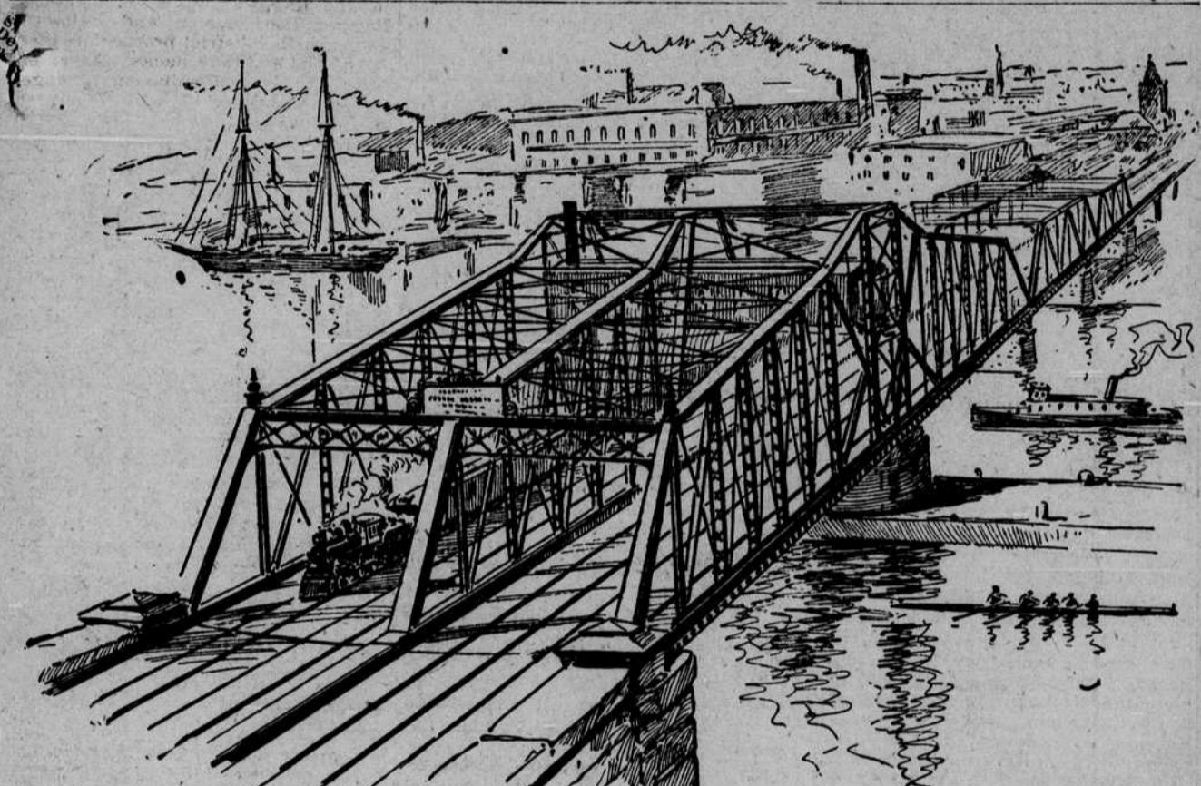
End View of the New York Central's new four-track steel draw-bridge over the Harlem River at 135th Street, Greater New York. The largest structure of its kind in the world.
