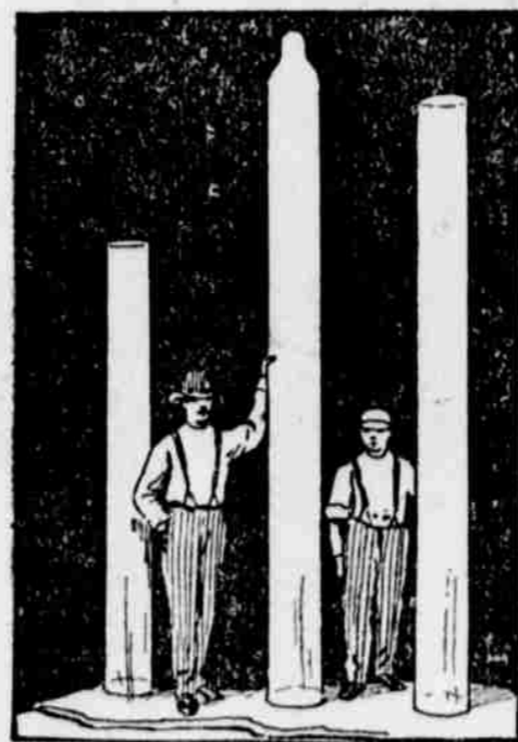
BLOWN BY MACHINERY.
