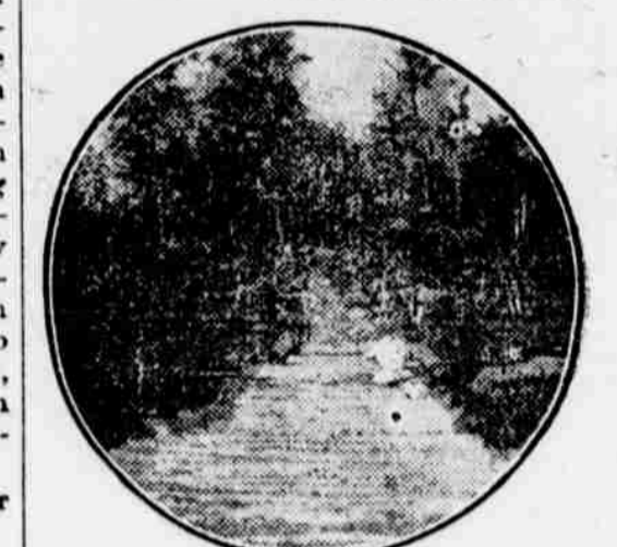
A CORDUROY ROAD IN THE TIMBER.
