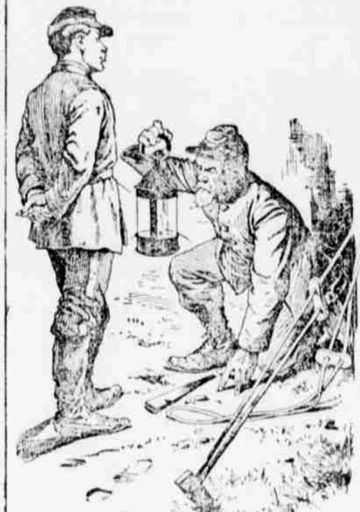
Was torn from the ground.
