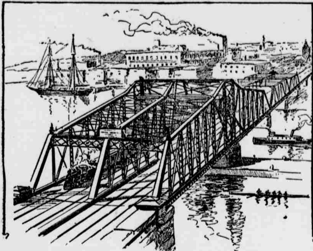
END VIEW OF THE NEW YORK CENTRAL'S NEW FOUR-TRACK STEEL DRAW-BRIDGE OVER THE HARLEM RIVER AT ONE HUNDRED AND THIRTY-FIFTH STREET, GREATER NEW YORK, THE LARGEST STRUCTURE OF ITS KIND IN THE WORLD.
