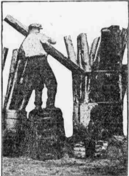
Removing Posts After Treatment in Creosote—The Posts Are Allowed to Drain in the Barrels.
