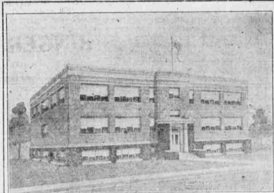
The above picture is a perspective of the exterior design of a modern Consolidated School Building.
