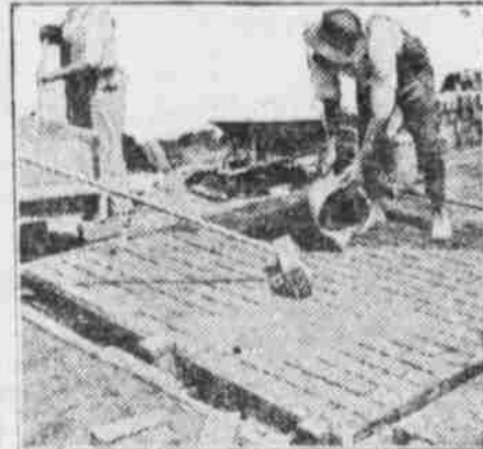
Laying Brick Pavement.
