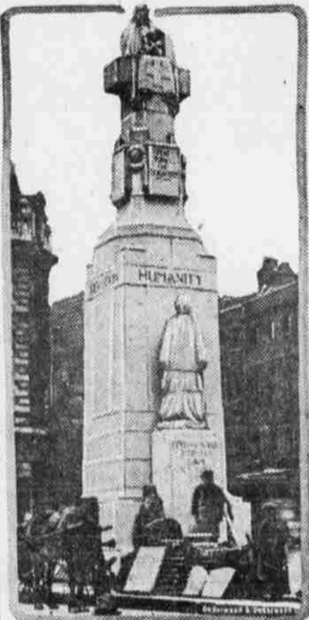
View of the new Nurse Edith Cavell memorial in London, with the scaffolding being removed. The statue of the nurse is still veiled.
