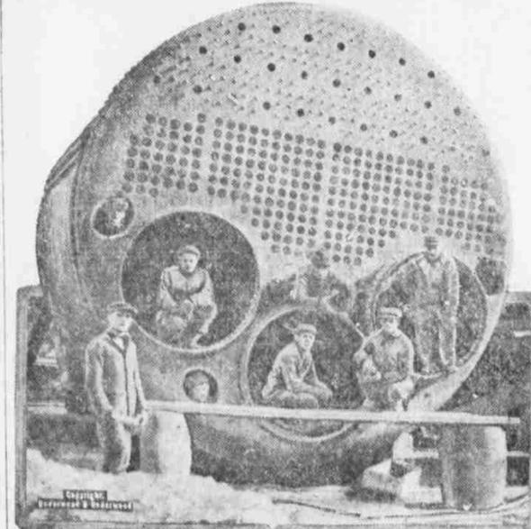
This boiler is one of six being built at shipyards in Chelsea, Mass. It has a diameter of 15 1/2 feet and its one-piece head is the largest ever made. The boilers weigh about forty tons each.
