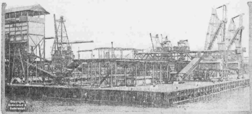
The coaling station at Cristobal, Panama canal zone, one of the largest in existence. Part of the coal is stored under water. Coal can be loaded here at the rate of 1,000 tons an hour.
