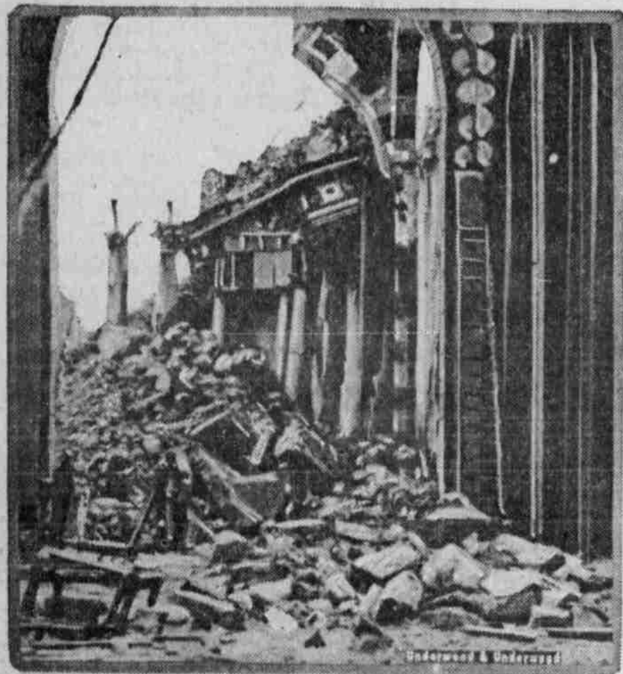
View of the ruins of the high altar in a church in the Mexican town of Teocelo, stricken in the recent earthquake.
