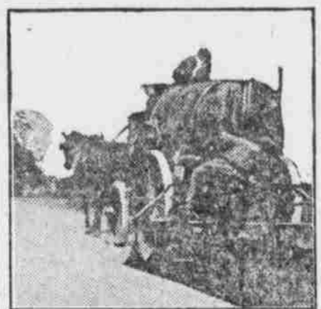
Surface Treatment of Macadam Road With Bituminous Material and Stone Chips.
