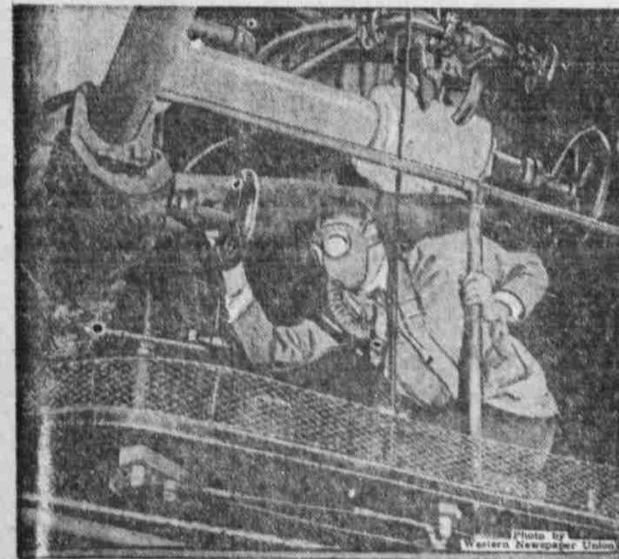
There are many industries where men work in the immediate vicinity of deadly gases, such as sulphuric acid, nitric, and hydrochloric acids, and the gas mask, slightly modified from its army design, is found an efficient preventive against injury from these fumes. Our photograph shows a workman repairing a break in an ammonia refrigerating plant, the mask protecting him from the noxious fumes.
