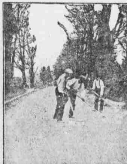
Making Necessary Repairs on Macadam Road.
