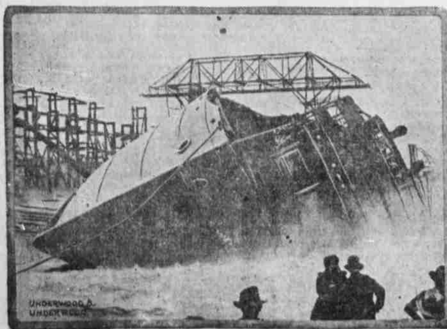
The Lake Fugard, an emergency fleet vessel launched at Buffalo, tipped to the extraordinary angle of 73.8 degrees and in seven seconds righted herself. A ship usually capsizes if it tips to an angle of 60 degrees. The Lake Fugard was launched with engines and everything else installed and steam up.
