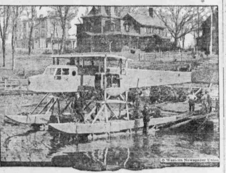
This huge seaplane is being built by the Witteman-Lewis Aircraft company, and is to be piloted by Capt. Hugo Sunstedt, a Swedish aviator, for a transatlantic flight for the \$50,000 Lord Northcliffe prize. The plane when rigged will have a wing span of 100 feet and a boat length of 72 feet. The boat is to be inclosed to protect against the cold and will carry three passengers besides the pilot. Its speed is 80 miles per hour and it is of the pusher | Tower will have to determine by caretype.
