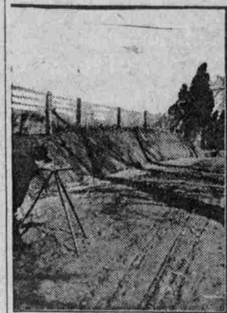
Getting Road Levels Preparatory to Improving Highways.
