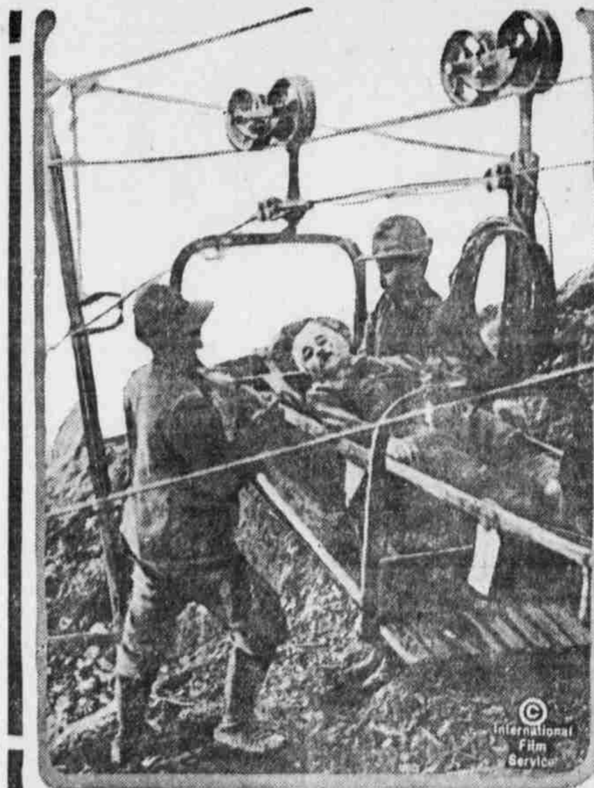
This photograph just received in this country gives an idea of the difficulties under which the Italian army fought the Austro-German forces on the Gorizia front. The wounded Italian soldier is being removed from a mountain peak position to the dressing station below by means of a cable railway.
