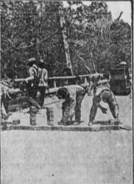
Laying Vitrified Blocks.
