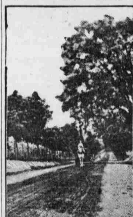
Road of Bituminous Macadam.
