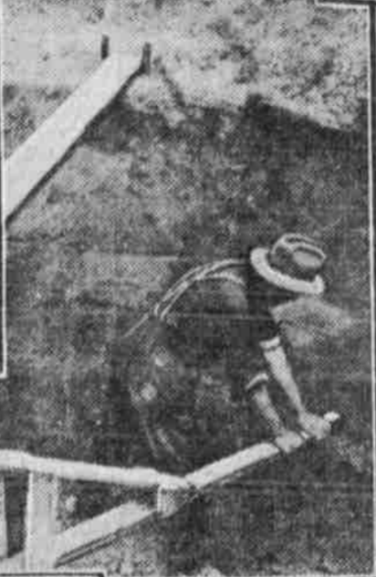
USING REAPER FOR TRIMMING SIDES OF SILO
