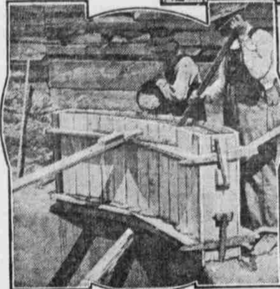
BUILDING UP SECTION OF SILO CURB
