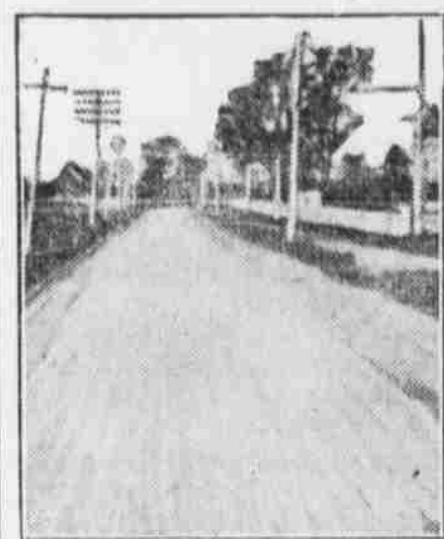
Good Road in Kansas.
