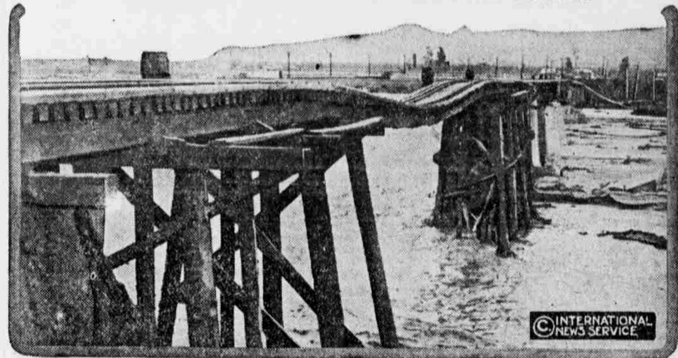
Floods in southern California are doing great damage and causing considerable loss of life. This photograph shows how the rush of waters wrecked the substructure of the railroad bridge over the Rio Hondo, making it impassable for trains.
