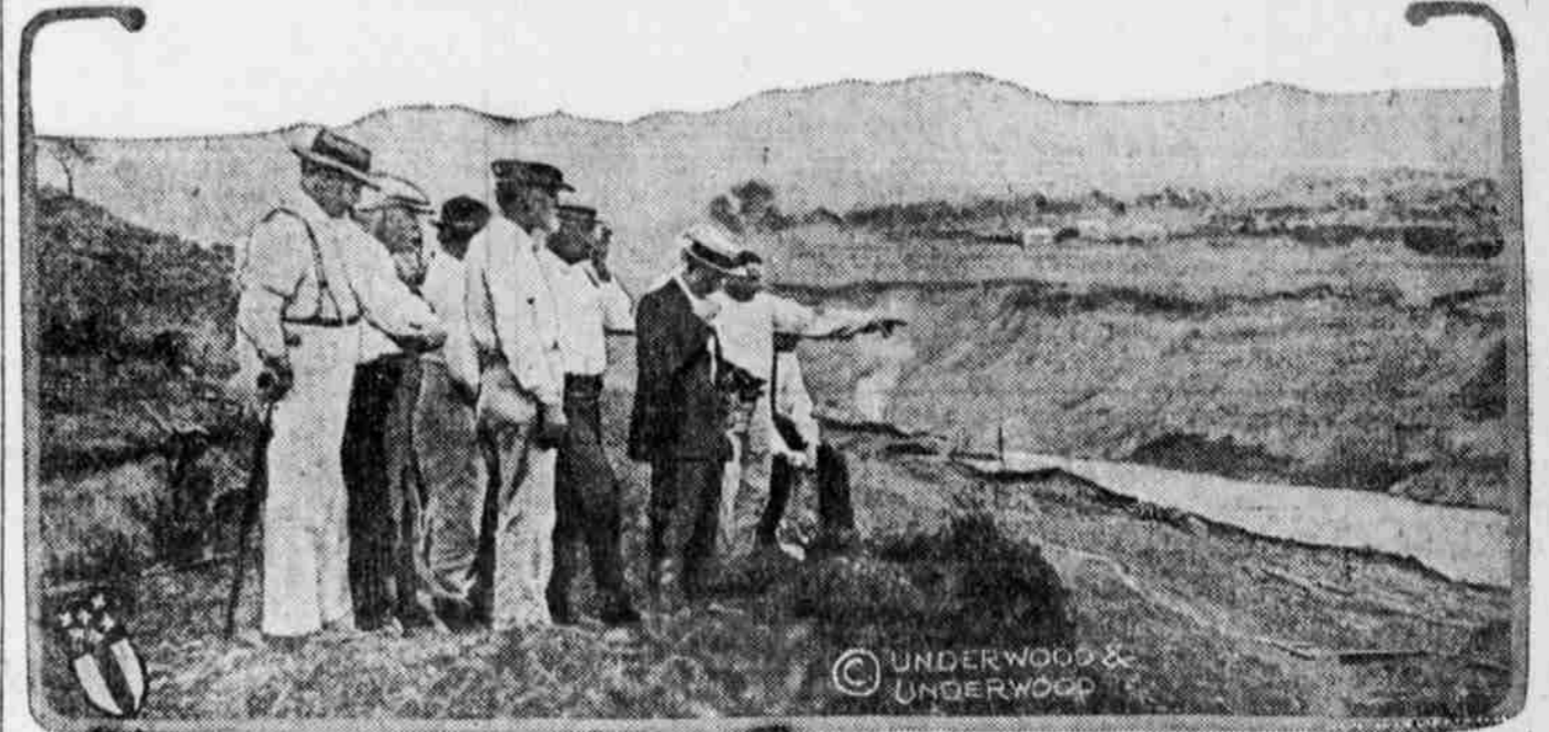
The great slides which have blocked the Panama canal have become a matter of such concern to the United States that President Wilson appointed a commission to study the causes of the slides. The photograph shows General Goethals and the commission viewing the slides and watching boats go through the canal.
