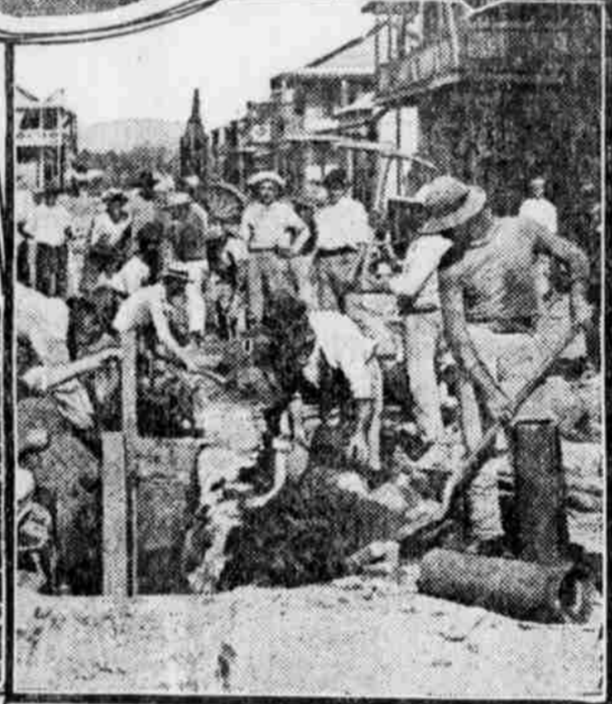
DIGGING SANITARY SEWERS IN CANAL ZONE
