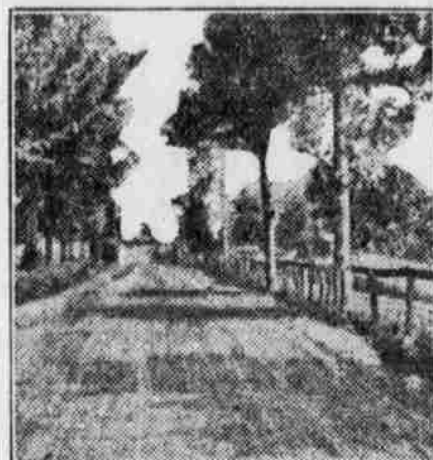
Macadam Road Treated With Asphalt Binder.
