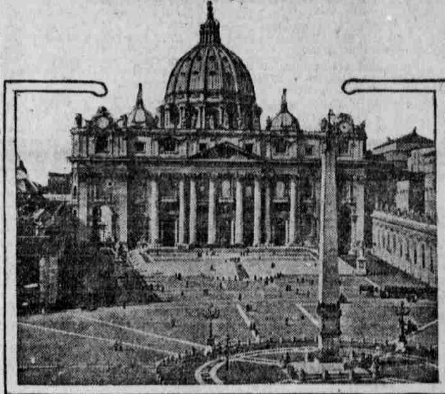
St. Peter's square in Rome was hard hit by the earthquake. The obelisk seen in the foreground in the photograph, was shaken and badly damaged; the famous colonnade, seen at the right, was lowered four feet, and the adjacent house, once occupied by the sisters of Pope Pius X, was seriously cracked.
