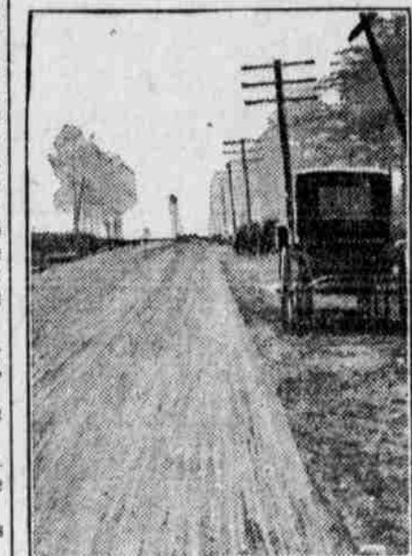
Road After Improvement With Top Soil Gravel.
