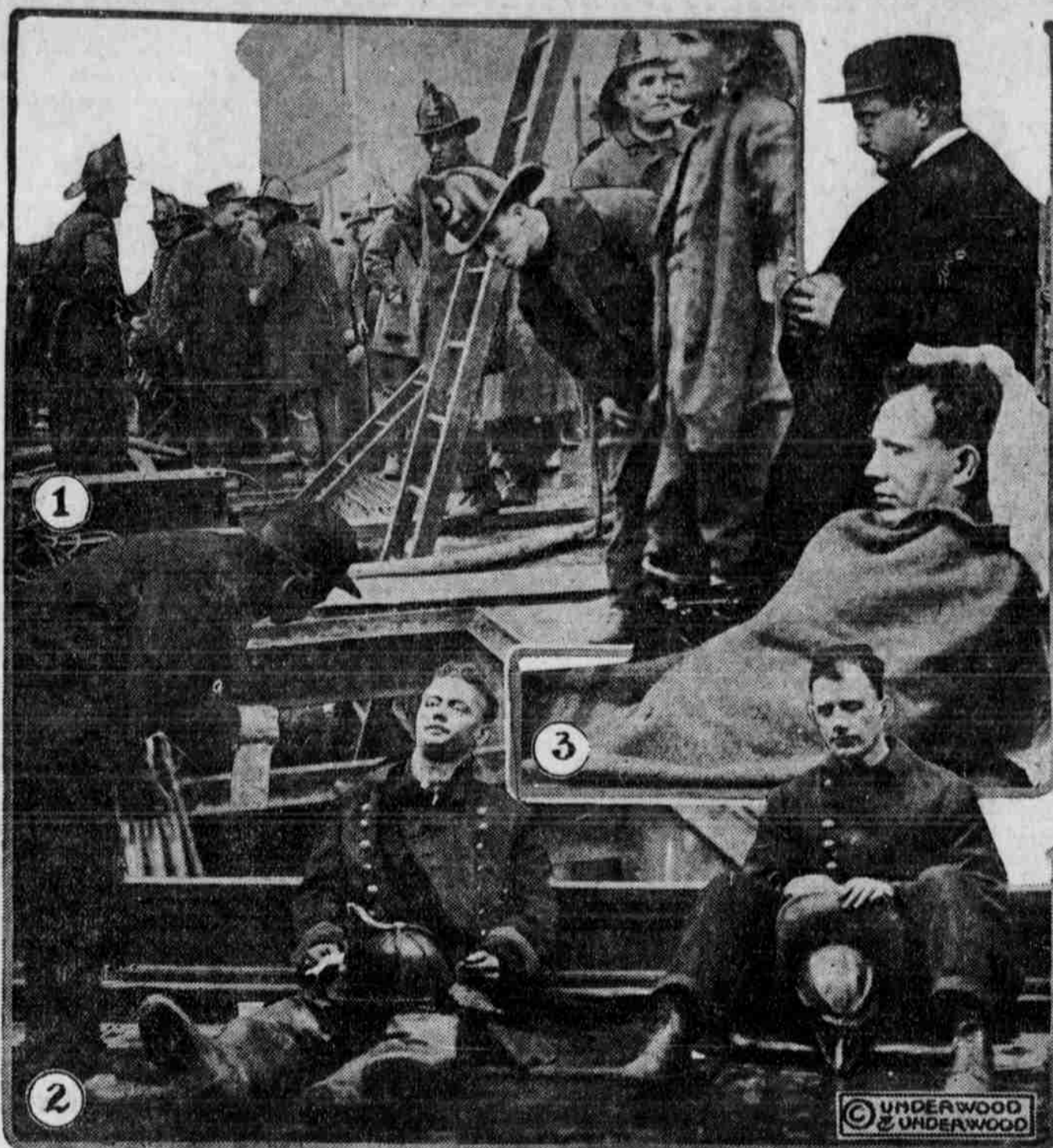
The burning of two large electric cables in the New York subway resulted in the partial asphyxiation of hundreds of passengers, and a panic ensued in which scores were injured. One woman was killed. 1. One of the gratings through which many passengers were rescued. 2. Firemen who were dragged to the street after being suffocated. 3. One of the overcome passengers lying on the sidewalk while a pulmotor is being prepared.
