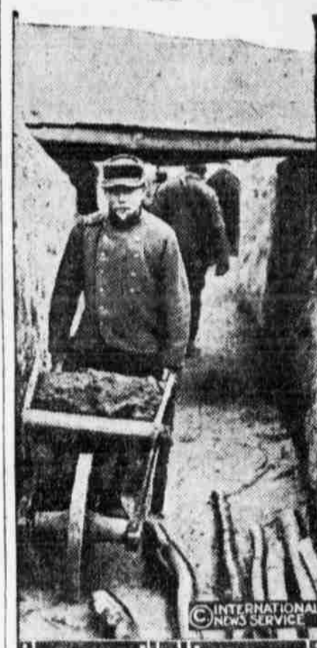
One of the deep trenches on the firing line in northern France. The allies have constructed hundreds of miles of ditches like this.
