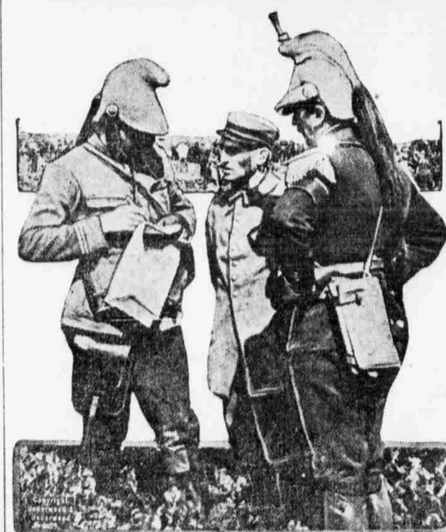
Just behind the firing line at Argonne this interesting little episode was photographed. Officers of the French general staff are interrogating a German prisoner concerning the strength and position of the Kaiser's forces.
