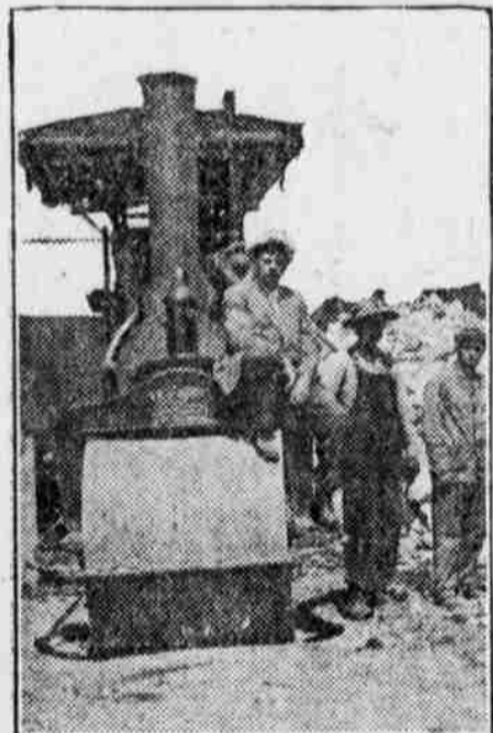
Rolling a Road Surface.
