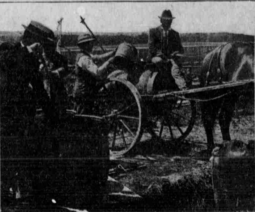
Getting the Spray Ready for Application.
