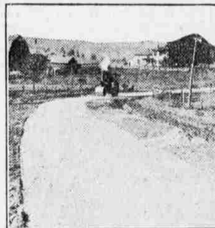
A Good Road in Wisconsin.
