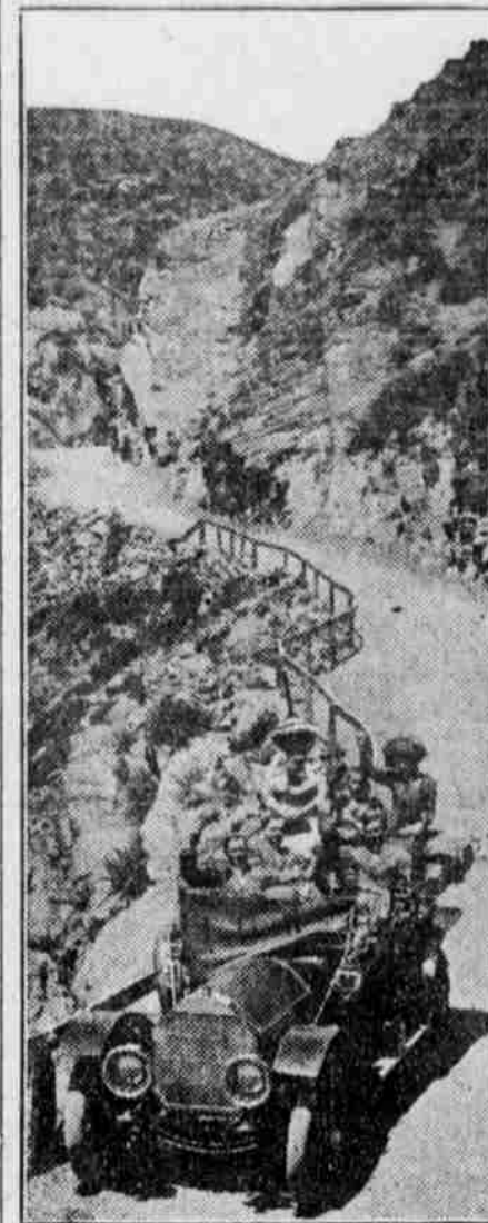
Entrance to Ute Pass, Near Manitou, Colo.—One of the Best Examples of Mountain Road Building in West.
