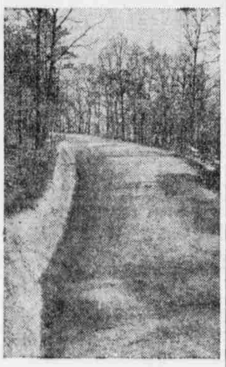
Same Road After Improvement.
