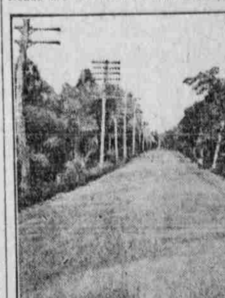
New York Cementitious Gravel Road.
