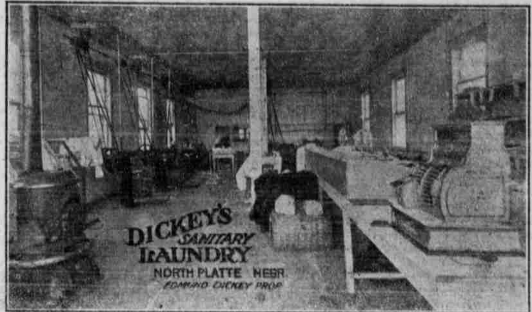
Interior View of Our Ironing Room
