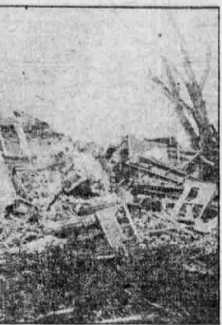
Wreck of home of Henry Figard. Barn was blown into house, but family escaped serious injury.
