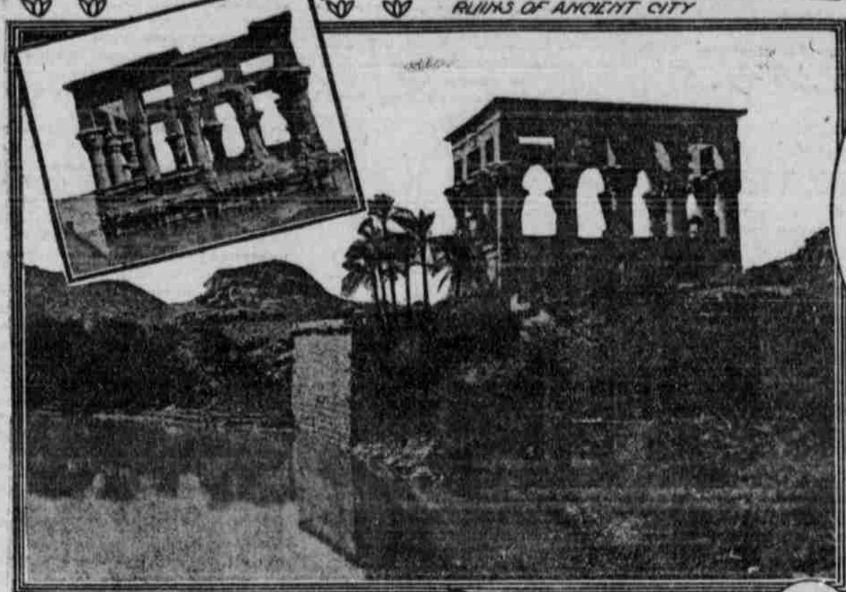
SHOWING HOW DAM HAS CAUSED NILE TO FLOOD ANCIENT TEMPLE
