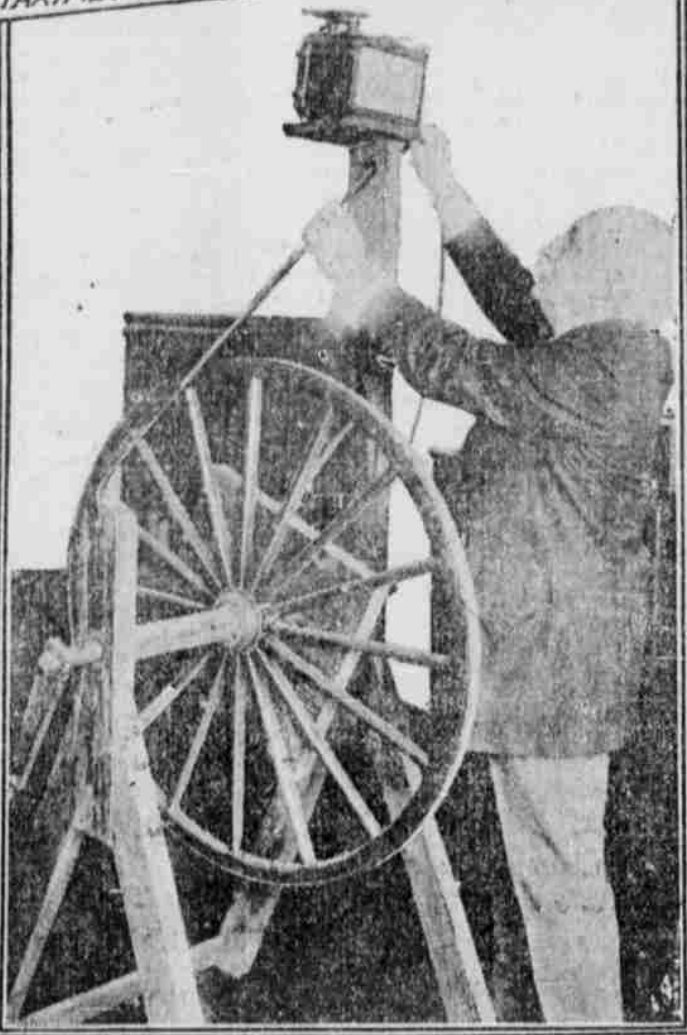
COL. HASKELL AND HIS FIRST MACHINE FOR TESTING TAXIMETERS
