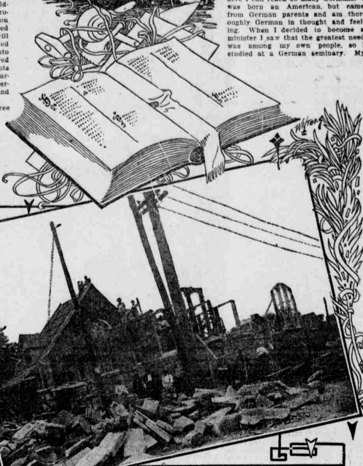
Beautiful Edifice Being Erected by Rev. Schwartz
