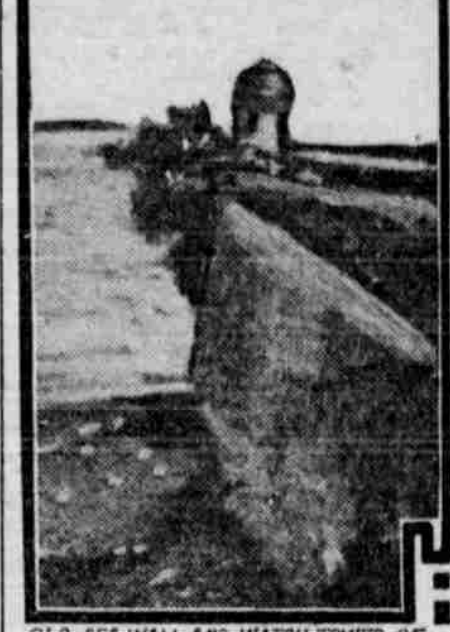
OLD SEA WALL AND WATCH TOWER OF THE CITY OF PANAMA
