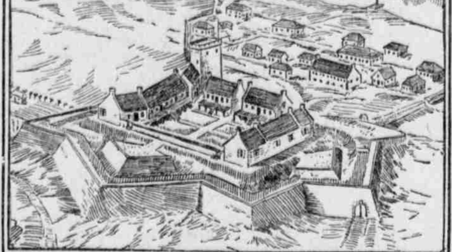
RESTORATION OF FORT TICONDEROGA
