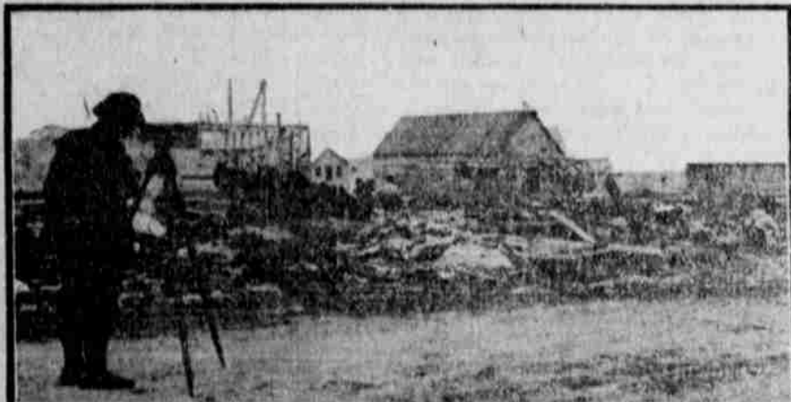
Ruins of Chisholm Hotel—Getting Lines for New Building.
