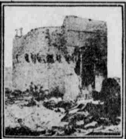
VAULT OF FIRST NATIONAL BANK
