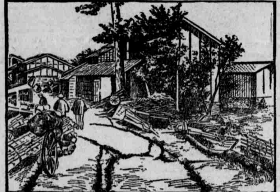
VILLAGE ROAD IN JAPAN, AFTER AN EARTHQUAKE.
