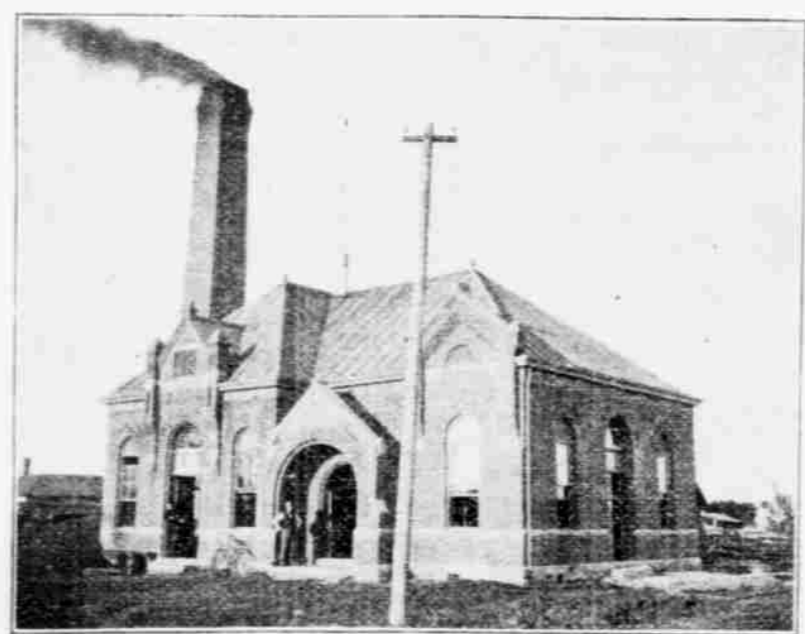
ELECTRIC LIGHT PLANT
